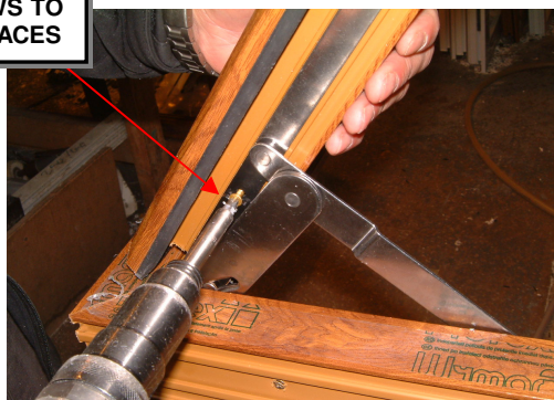
B) USING THE AJUSTMENT IN THE SLOTTED HOLES, ALIGN SASH AND FRAME BEFORE FITTING FINAL FIXING SCREWS
