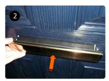
Insert the outer half into the aperture from the outside and hold in place while screws are inserted from the inside
