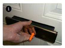
"nsert the inner half (with brushes) into the aperture from the inside.
