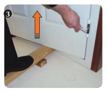
Use an air wedge (or similar) to lever and support the door at the correct height and tighten all screws to secure. Replace covers when finished.
