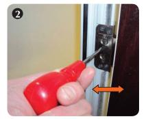
Insert a flat screw driver into the adjustment slot and lever the slide plate (B) in or out as required.
