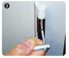
Back the screw off, using a 4mm allen key, at least 1 full turn. Only free off 1 hinge at a time unless you are adjusting the height at the same time.
